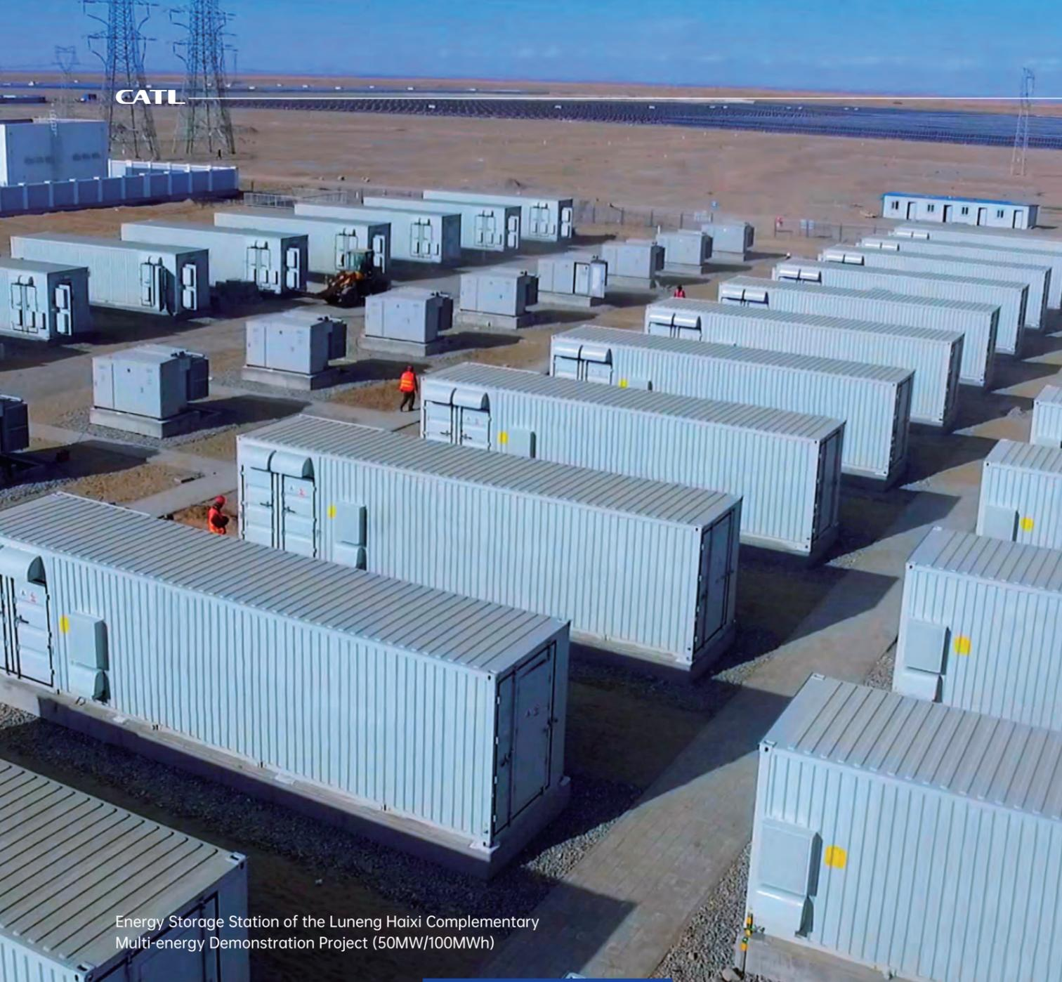
Energy Storage Station of the Luneng Haixi Complementary Multi-energy Demonstration Project (50MW/100MWh)
